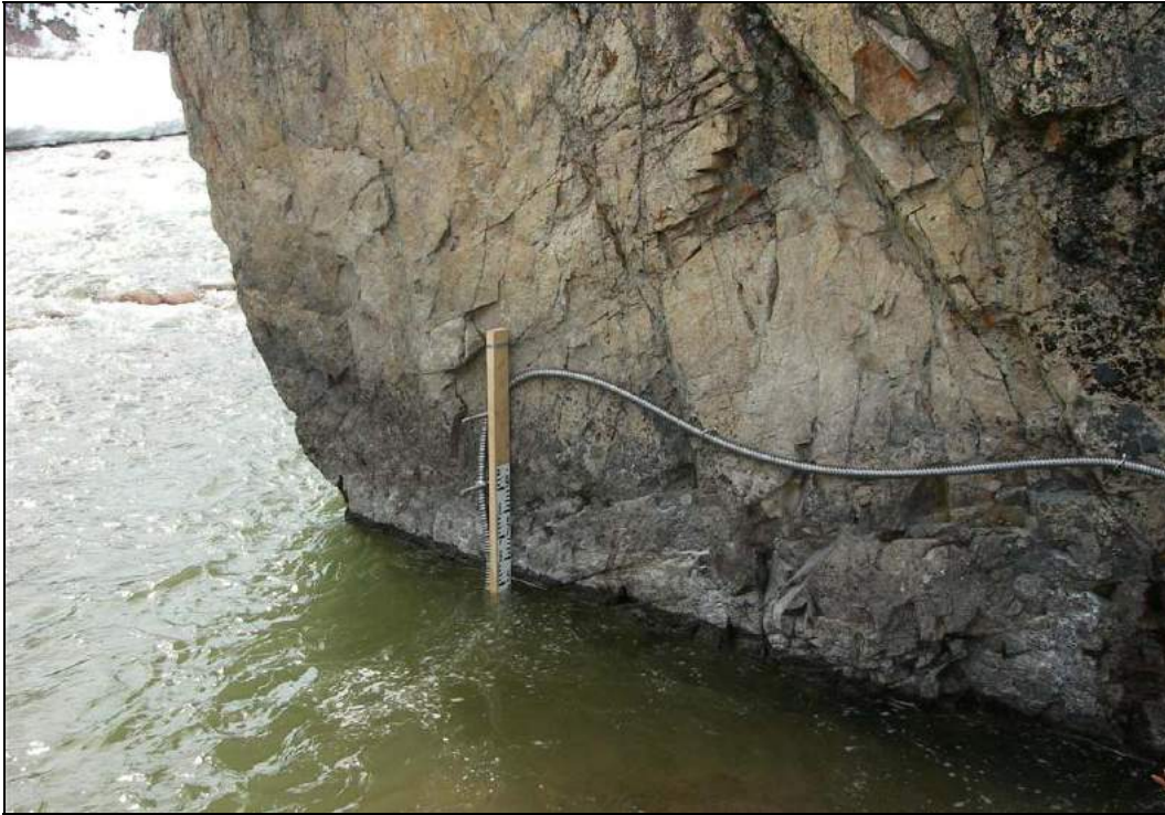
Plate 2.2-1. SCTR-2 automated hydrometric station, newly installed in 2007.
