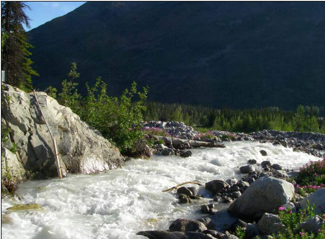
Plate 2.2-2. SCTR-3 automated hydrometric station, newly installed in 2007.
