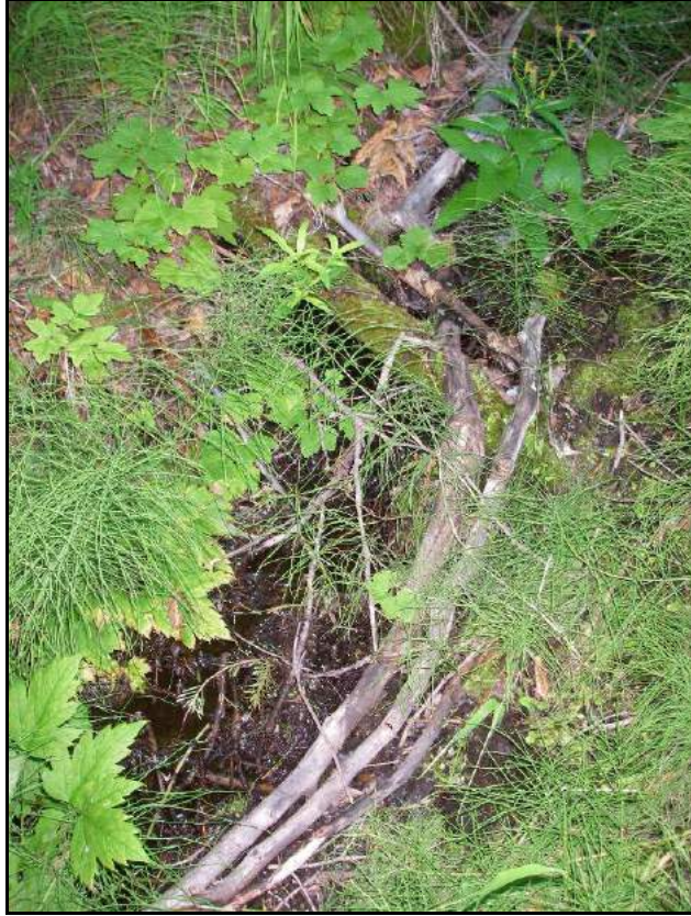
Site 183 – Downstream seepage
