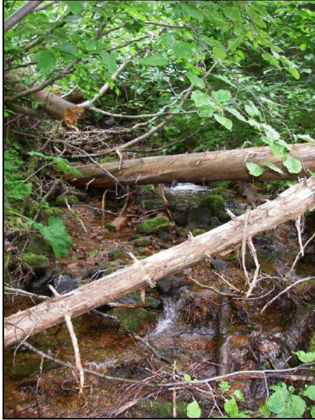
Site 198 – Upstream, showing some scour
