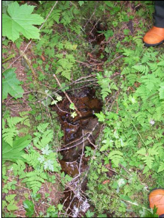
Site 138 – Upstream view, seepage
