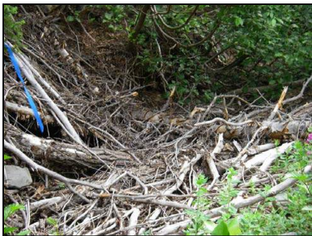
Site 300 – Abandoned channel
