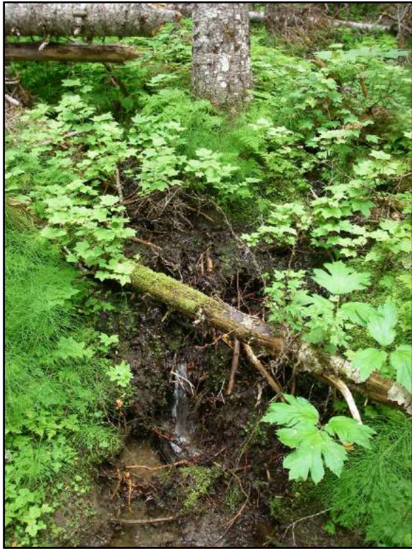
Site 234 – Upstream seepage barrier
