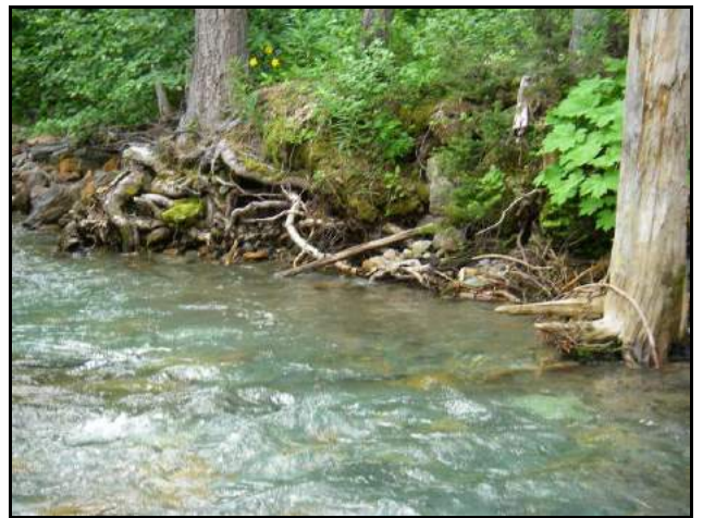
Site 300 – Erosion right bank
