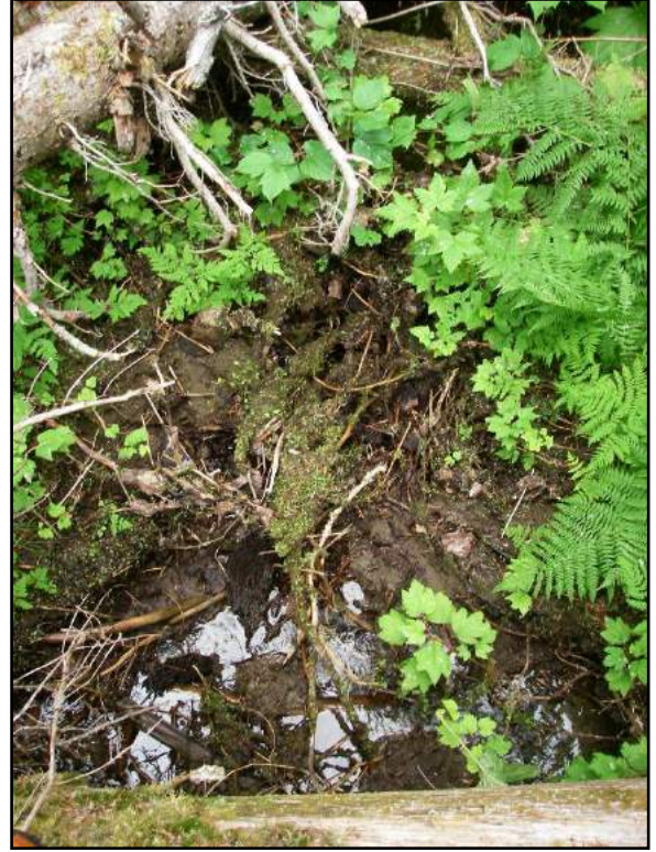
Site 234 – Downstream view, almost a seepage
