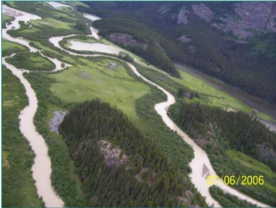
Figure 25.25 Mess Creek Flood Plain Road Centreline Crossing
