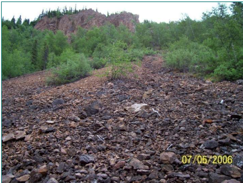
Figure 25.28 Tallus Slope along Lake Shore near km 22.0
